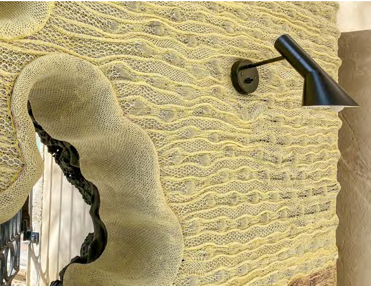
Fig. 15. Interior textile and fittings, Meristem Wall.
