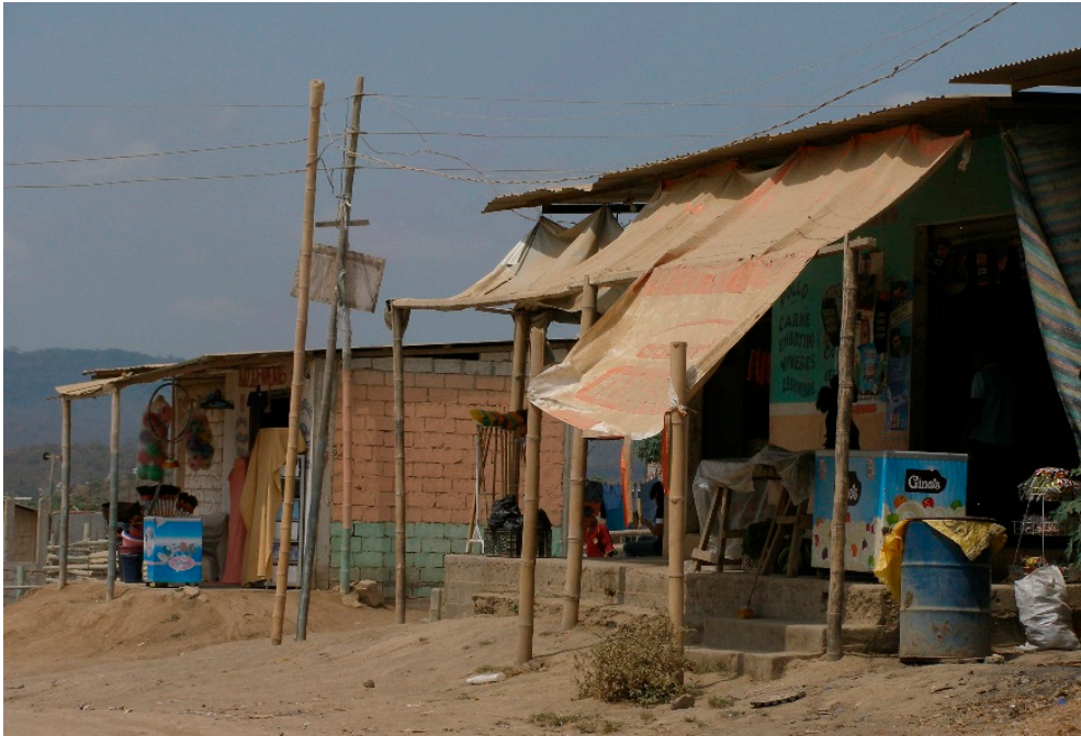
Figure 19. A street in the Sergio Toral neighbourhood, with informal shops facing a main street.
