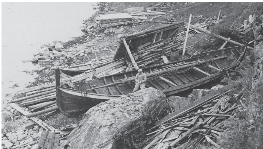
Figure 12.1. Bernhard Færøyvik measuring a larger Åfjordsbåt known as a fembøring in 1936. The thorough documentation work conducted by Færøyvik and others during this period allowed for the survival of the Åfjord tradition and informed the construction of the boats used in this study. Photograph by Kristian Kielland, Norwegian Maritime Museum, Id: NSM.1701-161.
