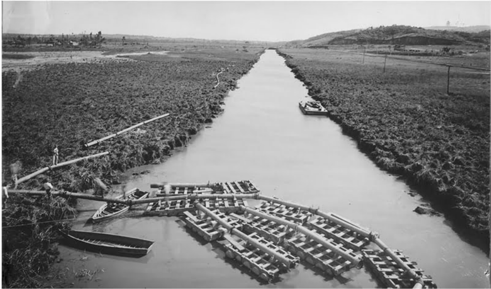
Figure 6.2: Straightening of the Pinheiros River: first cut of the canal, southwards from Cidade Jardim Avenue. Workers are visible on the left riverbank. 1936. Source: [116].
