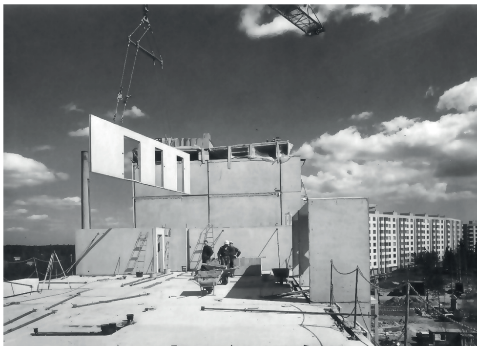
Figure 4 Assembly of prefabricated wall elements in a house-building project in the Million Homes Programme (Marmstål and Nordberg, 1992).
