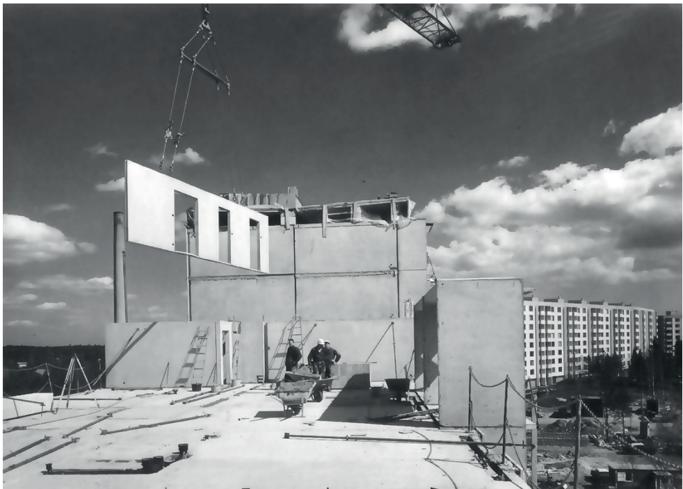
Figure 4 Assembly of prefabricated wall elements in a house-building project in the Million Homes Programme (Marmstål and Nordberg, 1992).
