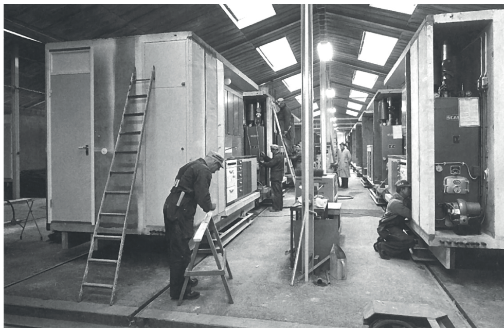
Figure 5 Factory production of volume elements including a complete kitchen, bathroom and service installations, around 1960 (Marmstål and Nordberg, 1992).
