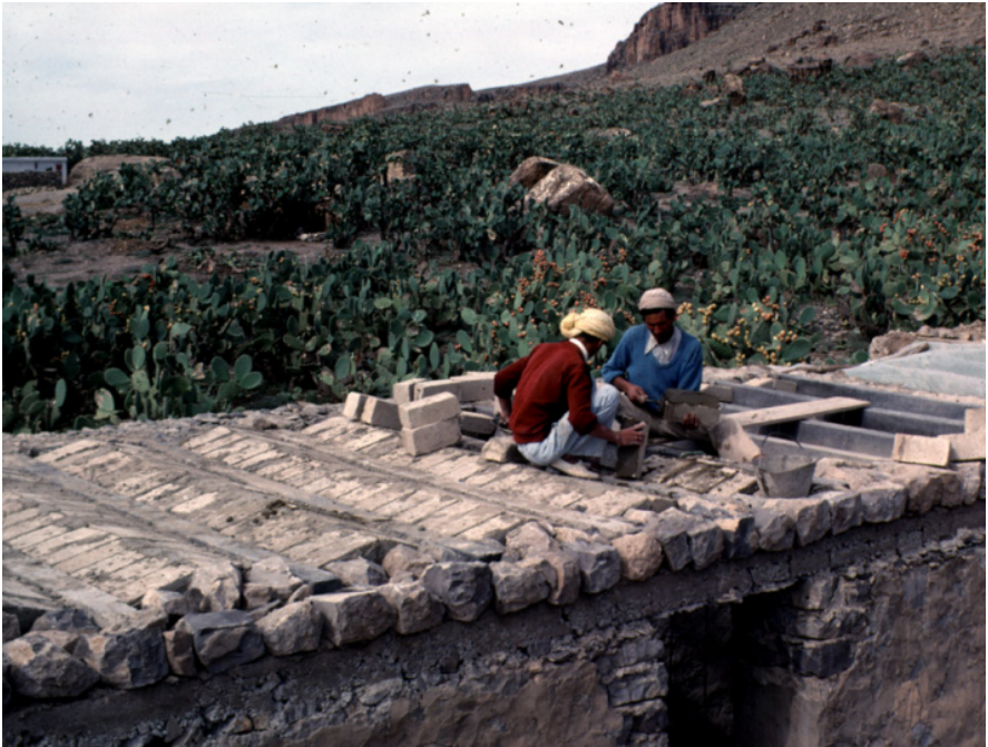
Figure 4: Construction of flat roof by self-builder with instructor Source: Johnny Åstrand, 1981
