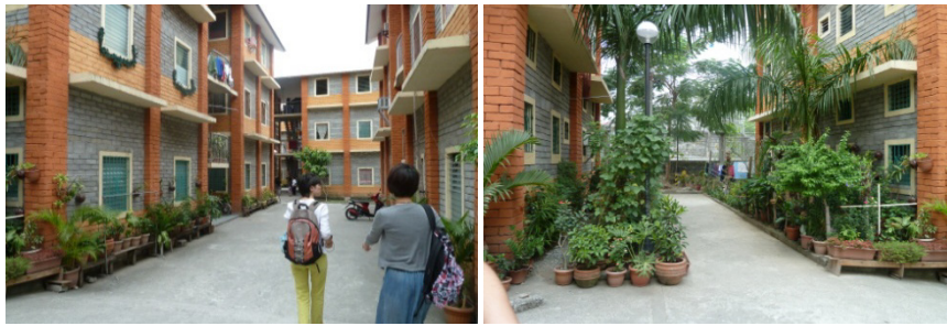
Figure 4.2 Taguig project is the first medium-rise building for OSHH implemented by Habitat for Humanity Philippines, households and volunteers. A three storey building in which each apartment units consists of two levels; the first level is for living and wet chores; the second level provides space for a loft for sleeping. Photos: Alvaro Vásquez-Esparza, Field trip to The Philippines 2011
