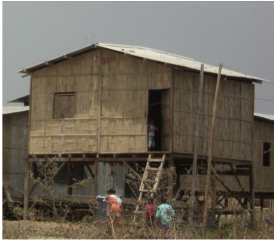
Figure 5. Hogar de Cristo Bamboo house where the structure is made in wood and the walls are pre-fabricated bamboo panels. The design is based on the vernacular house of the Coastal Region in which the second storey is elevated 2,40 m from the ground floor to allow for shaded outdoor activities. Photo: Ivette Arroyo, 2011
