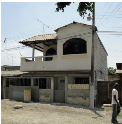
Figure 10. New housing replacing first housing typology in phase 3 with reinforced concrete structure and masonry block walls. Photo: Ivette Arroyo, 2009
