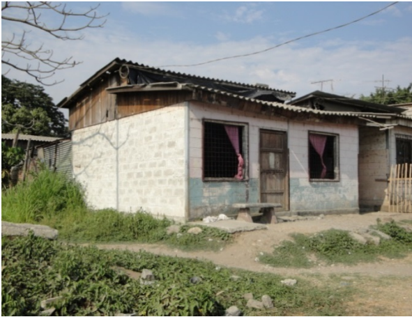
Figure 6. First housing typology for phases 1 to 6 where the construction system consisted of clay block walls and metal framework.
