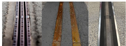
Fig. 2. Illustration of different road-bound conductive ERS solutions.
