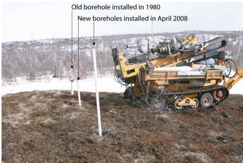
Figure 3 Two new boreholes were installed at “Kursflaket” in spring 2008 close to the borehole installed in 1980 (Photo: J. Åkerman).
