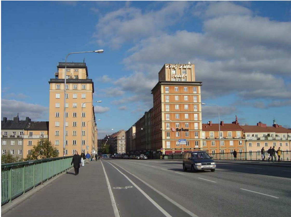
The bridge "St Eriksbron" towards Birkastan
