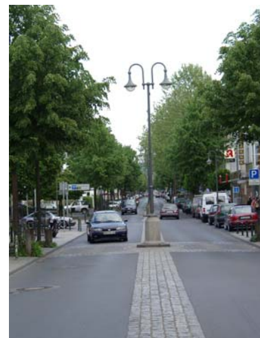
Narrower running carriageway – suitable where place status is high relative to link status
