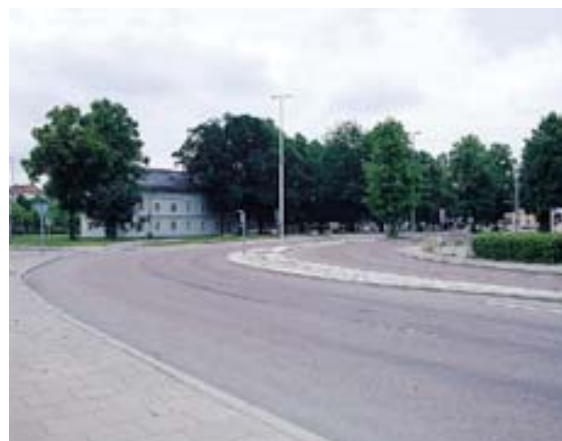
Before situation at the stretches
