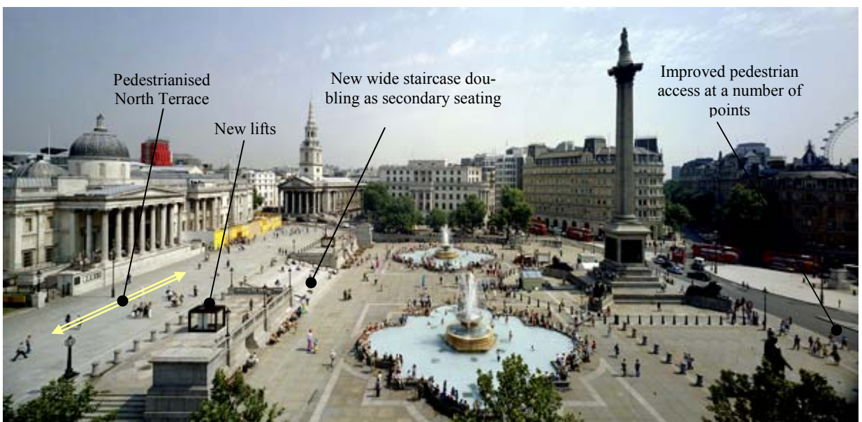
Trafalgar Square after reconstruction – North Terrace was pedestrianised, now acting as better pedestrian link in the area and connecting the National Gallery to Trafalgar Square. The new space reinforces Trafalgar Square's status and value as a 'World Square'.
