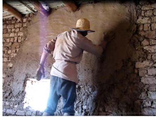
Figure 5.31 Plastering layer is smoothen by wet hand.
