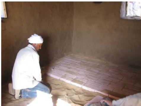
Figure 5.34 Floor making using sand tiles.
