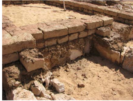
Figure 5.22 Lime is mixed into the footing mortar.
