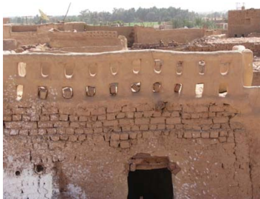
Figure 4.50 Example of exterior fences (parapets) in the roof floor made from mud brick .
