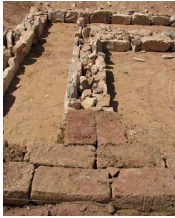
Figure 5.21 The stone and brick footing.
