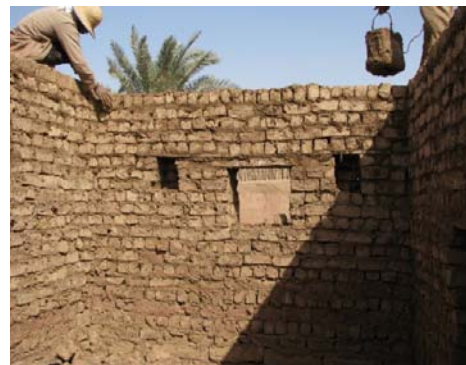
Figure 5.24 Windows and niches during wall construction.
