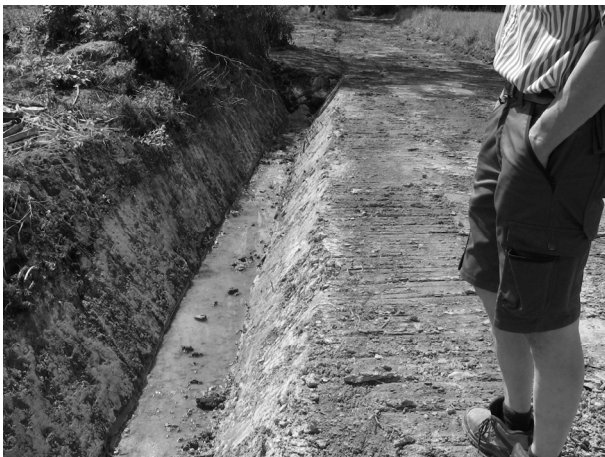
Figure 44. New Ditch in line with Piped Ditch (Fig. 43)
