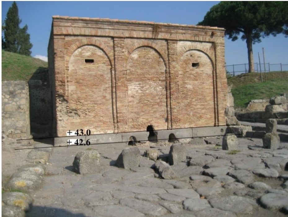
Figure 2.2. South façade of Castellum Aquae with indications of levels for the three openings. The middle one slightly above and the left and right ones are on the same level. Photo and indication of levels by author.
