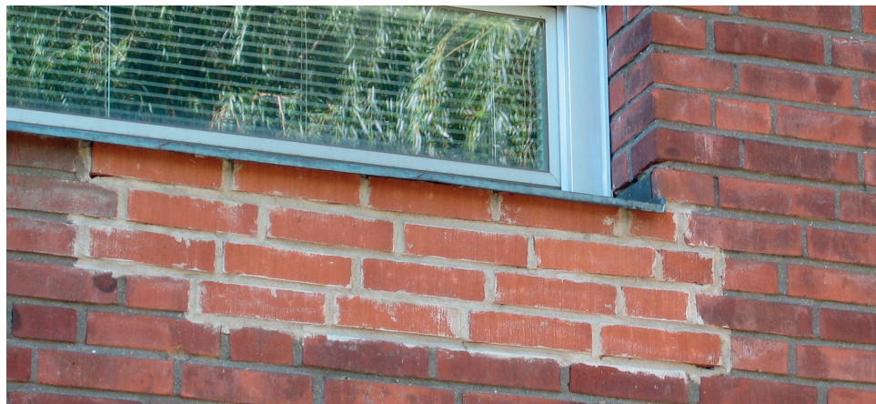
Figure 2. An example of adverse effects of selecting unsuitable mortar and shoddy workmanship on repointing
