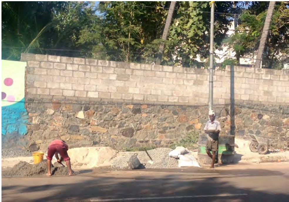
Figure 16. Cement workers in Kerala, south west India, handling wet cement.
