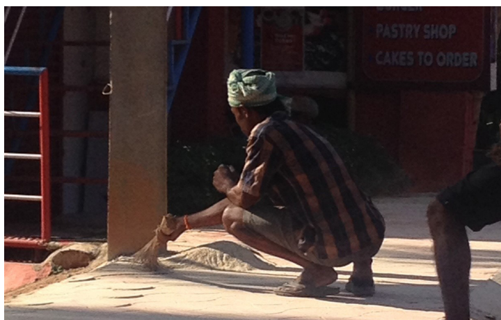
Construction worker, Kerala South west India.
