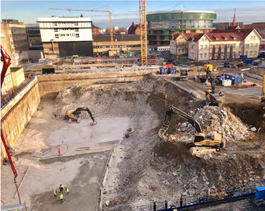
Figure 38. Further preparation work, Skane University Hospital, Malmö.
