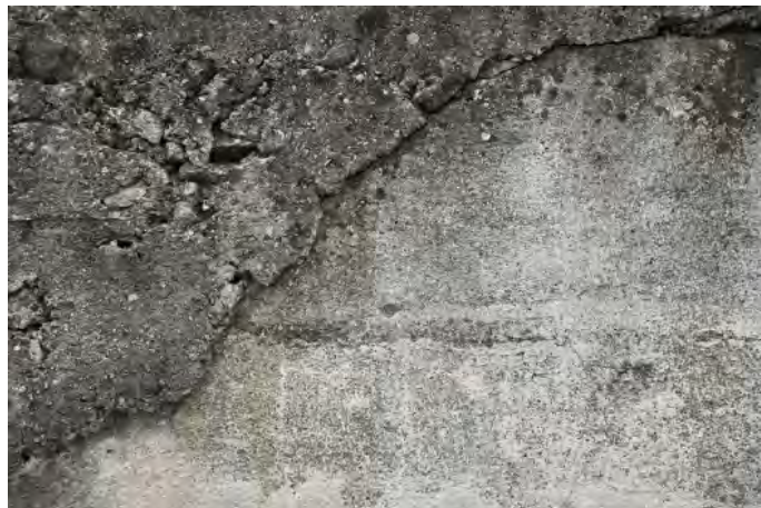
Figure 19. A concrete wall. (Photo: Pixabay)
