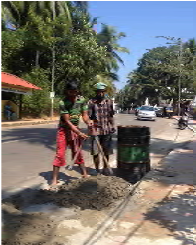
Figure 17. Cement workers in Kerala, south west India.
