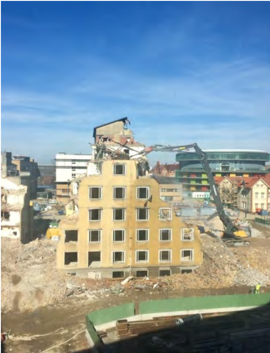
Figure 36. The demolition of old concrete building at Skane University Hospital, Malmö.
