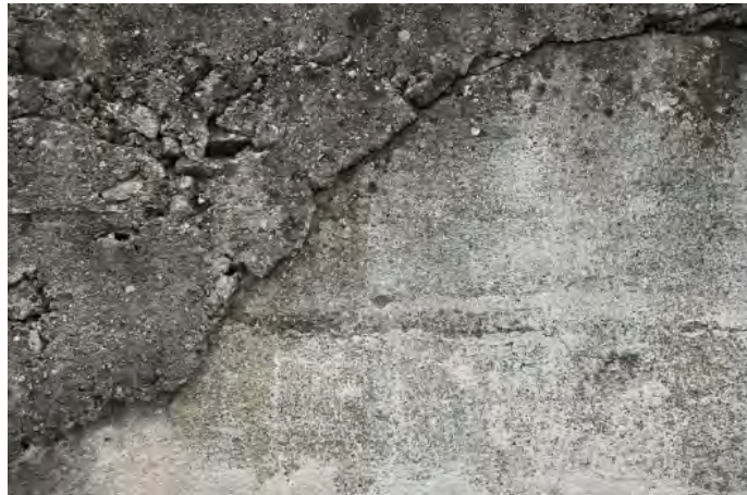
Figure 19. A concrete wall. (Photo: Pixabay)
