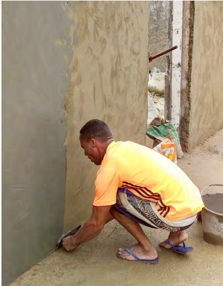
Figure 43. Construction worker, Paqueta, Brazil.
