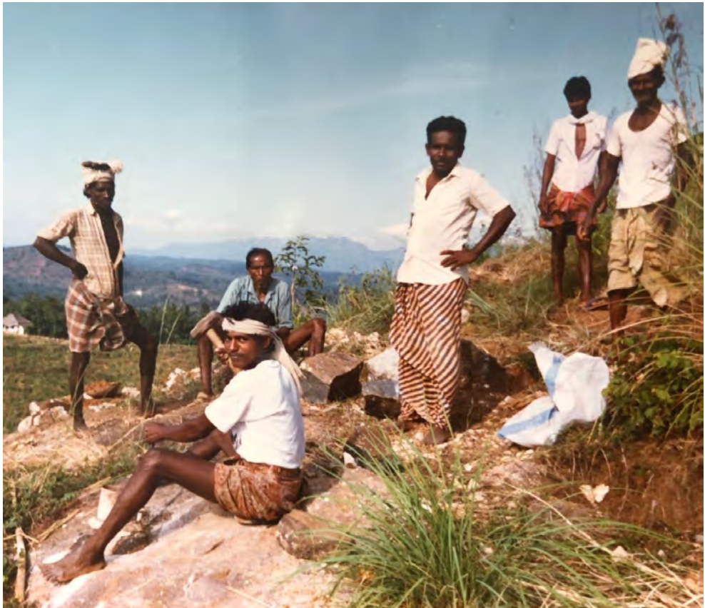
Figure 2. Construction worker team, Kerala, south west India.
