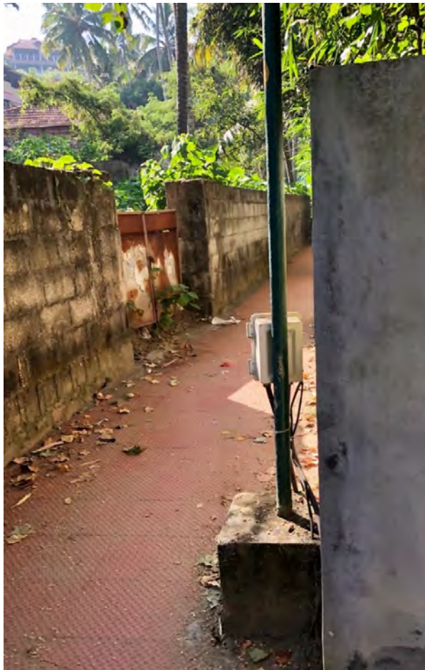
Figure 20. Cement bricks and concrete walls, Kerala, south west India.
