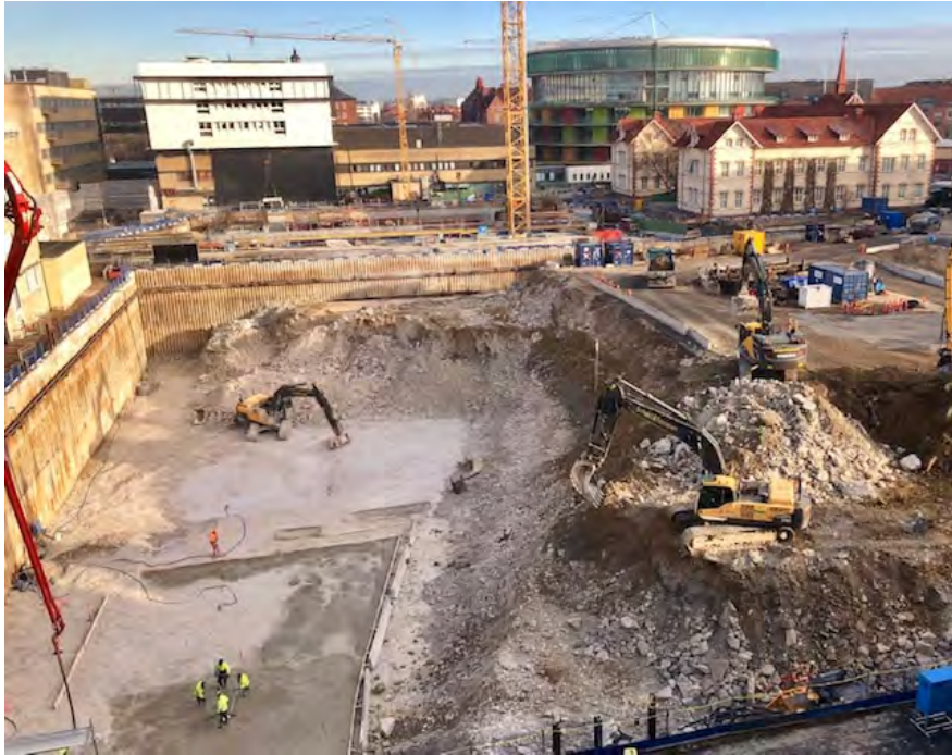
Figure 38. Further preparation work, Skane University Hospital, Malmö.
