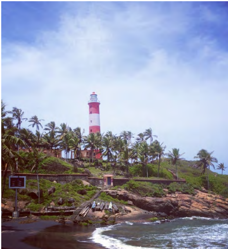
Figure 21. Lighthouse and wall built with bricks and stones, respectively, and mortar, Kerala, south west India.
