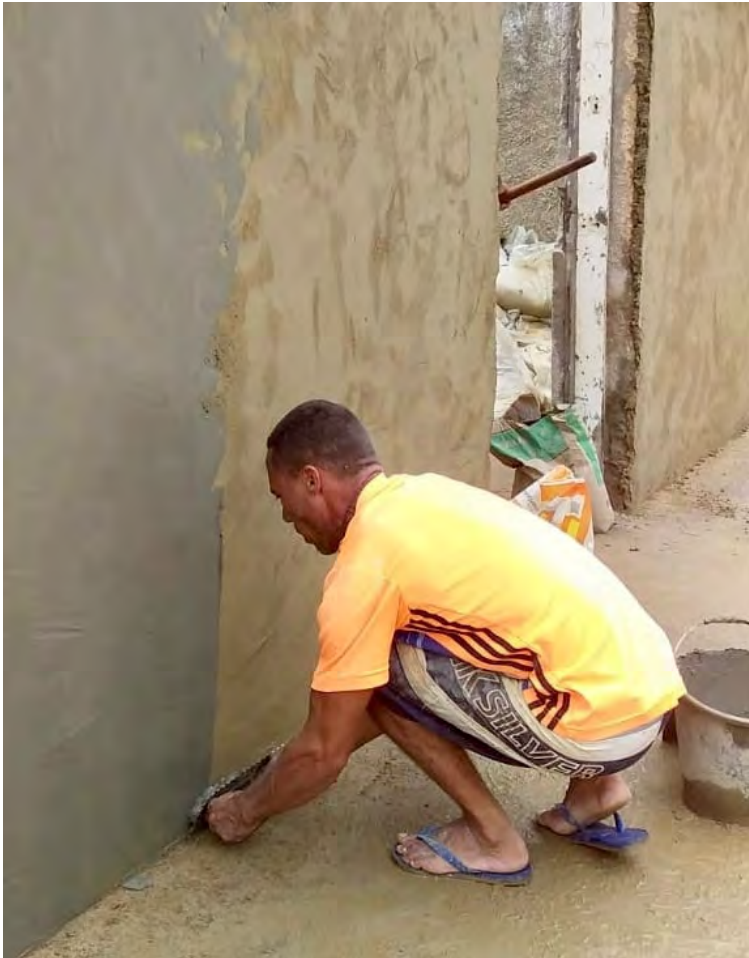
Figure 43. Construction worker, Paqueta, Brazil.
