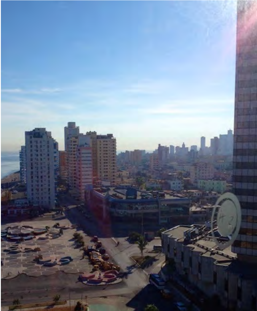
Figure 27. Concrete is used in buildings and car parks, Havana, Cuba.
