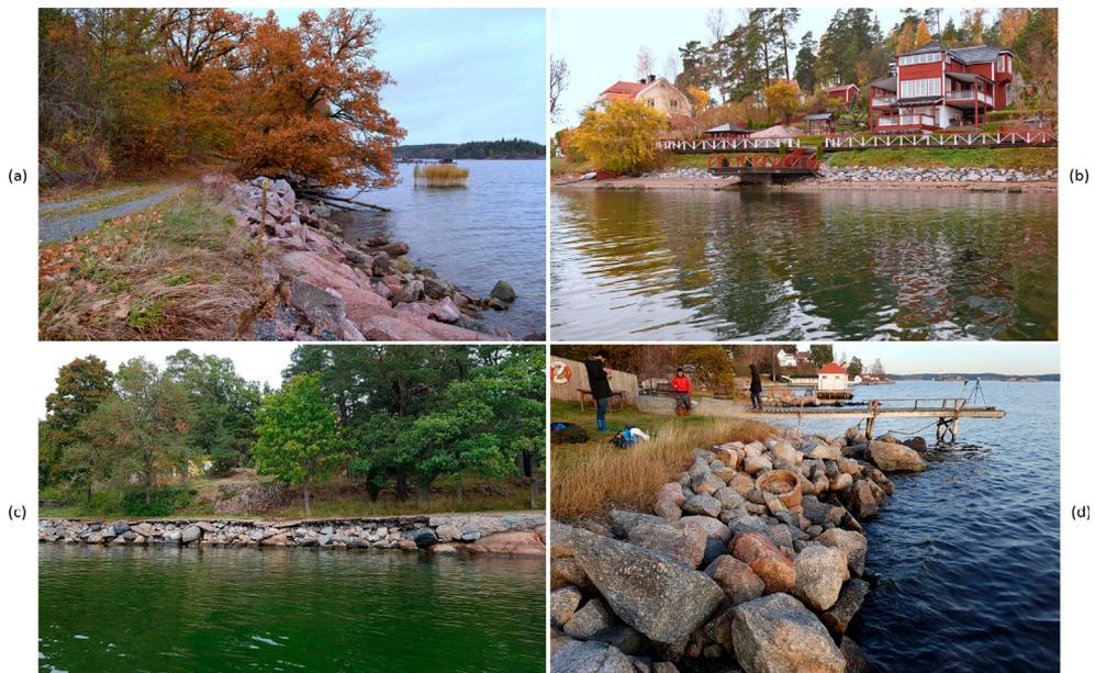
**Figure 3-9.** Examples of landowner initiative of erosion protection along the Furusund Fairway. (a) A rip-rap revetment is protecting a private road. (b) A seawall of rocks stabilizing the shoreline in front of a house. (c) A seawall that have been damaged by wave forces. (d) A rip-rap revetment protecting private property from eroding. (Photos taken in October 2016 (a-b), in August 2019 (c), and in December 2019 (d)).
