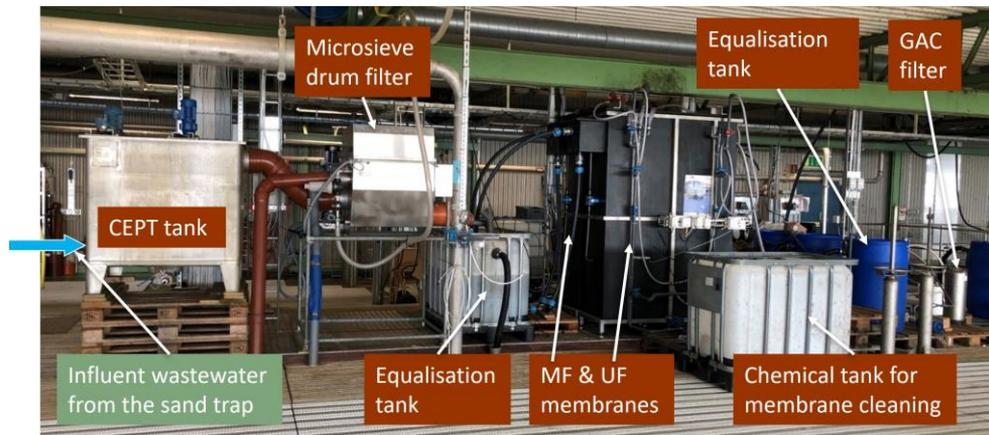
**Figure 8.** The pilot-scale treatment plant employing physicochemical processes at Svedala WWTP.
