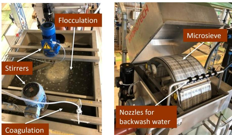
**Figure 9.** Coagulation and flocculation in the CEPT tank (left) and the drum filter used for microsieving (right).
