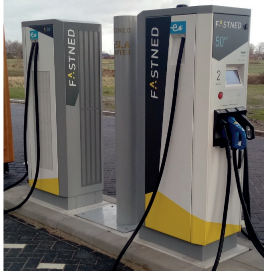
Figure 1.3: A DC fast charger [12].
