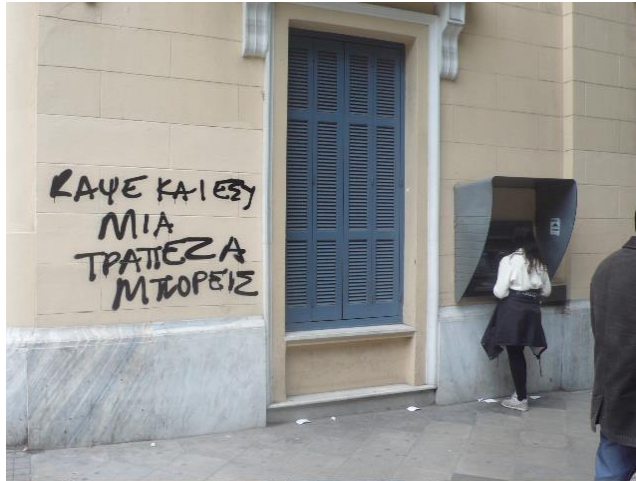
Figure 10 BURN A BANK YOU TOO; YOU CAN DO IT , Plaka, Athens
