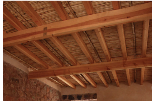
Figure 6. Roof structure developed based on roofing vernacular techniques in Saint Catherine. (Credits: Nashwa Ibrahim).
