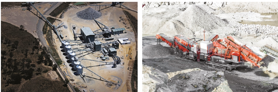
Figure 1.6 Typical stationary C&S plant (left) and a mobile C&S plant (right).
