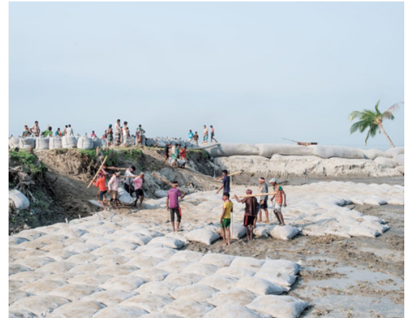
Sandbags being laid for the foundation of a river bank defence, at Elisha Ferry Ghat, on the bank of the Meghna river on Bhola Island, Bangladesh where as much as 18% of the country's land mass could be inundated by sea level rise.
