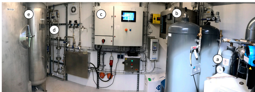
Figure 10. Photograph of the pilot-scale ozonation plant. Showing the oxygen generator units (a), ozone generator (b), control panel (c), ozone injection points (d) and reaction tanks (e).
