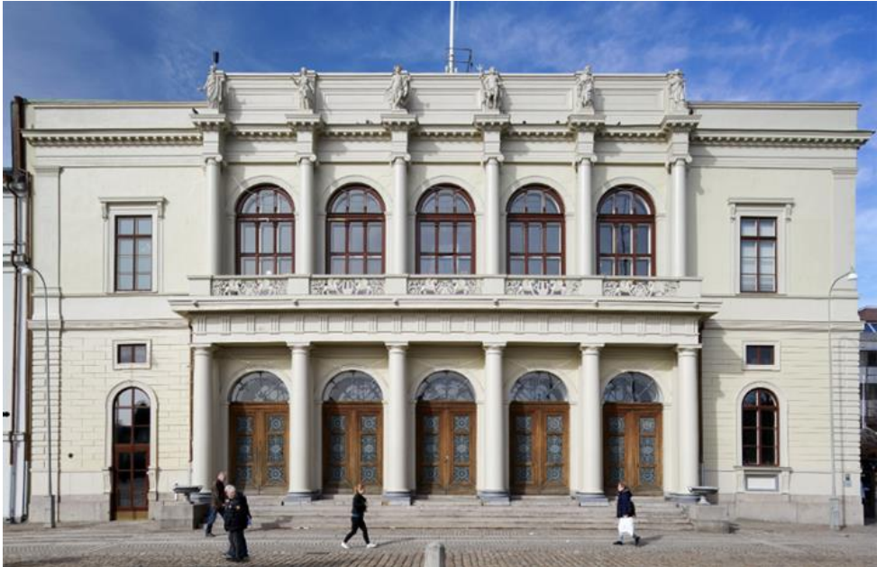
Figure 7: Users are no longer separated when entering this old public building. A new entrance, on the same level as the square, is located to the left of the steps.
