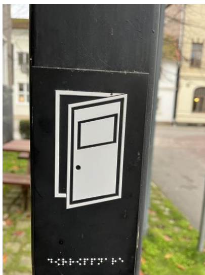
Figure 8: Many door openers are marked with a wheelchair symbol, but here it has been preferred to show what happens if you press the button: the door opens.
