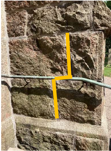
Placering fogbruk 5: hydraulisk Gotlands kalk.
