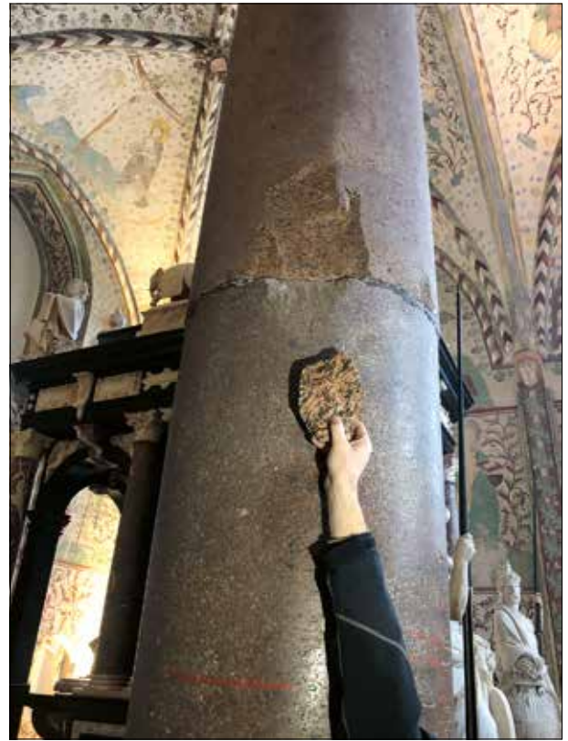
Fig. 9. The bedrock used for the King's Pillar in Roskilde Cathedral is very like the stone sample taken from the boulders in the forest at Djurröd. Photo: Chatarina Ödman 2022.
