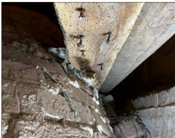
Fig. 6. The easternmost tie beam of the Gloslunde nave. It is partially built into the vault. On the underside of the beam there are fragments of pine boards, built into the vault, with traces of red and white paint. Photo: K.-M. Melin 2023.
