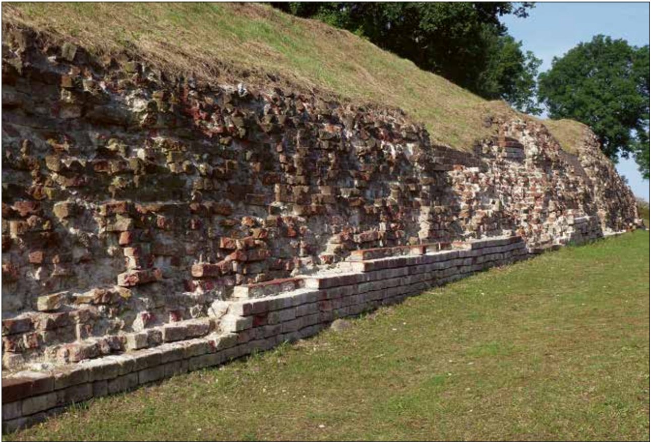
Fig. 1. The main wall of Danevirke, strengthened with fired bricks. Photo: Holger Ellgaard 2014. CC BY-SA 4.0
