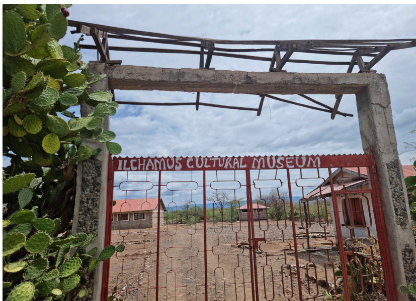
Image 24. Il Chamus Cultural Museum main gate. After several years of abandon, signs of neglect are starting to show: the exposed brickwork around the gate is crumbling, the grass thatch has fallen out of the awning and the cactus fence is starting to grow over the gate (own photo).
