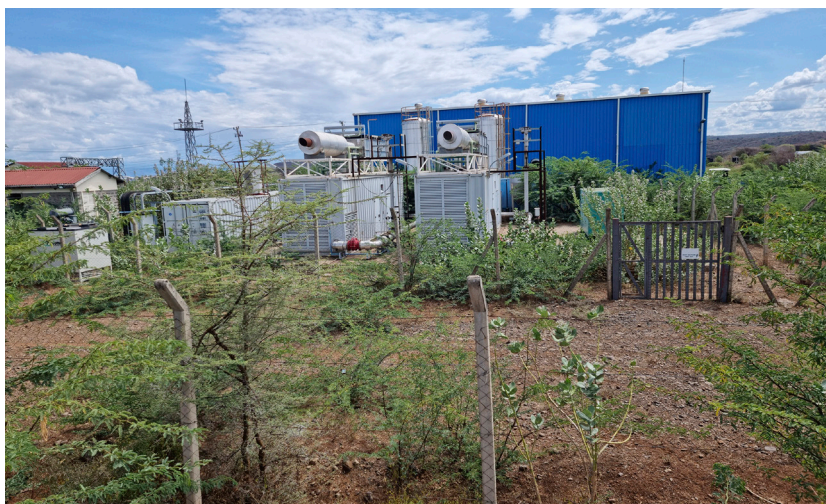
Image 28. Cummins Power Generation plant sits atop the hill above Marigat, waiting to be fed with Prosopis logs to convert into electricity. The plant was built near a national grid substation so the electricity produced could easily feed into the national system (own photo).
