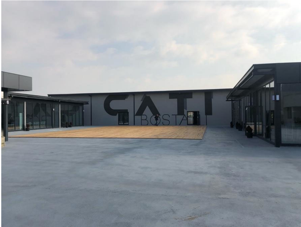
Figure 2. The exterior and roof-top entry to Çatı gallery. Photograph: Torsten Janson.
