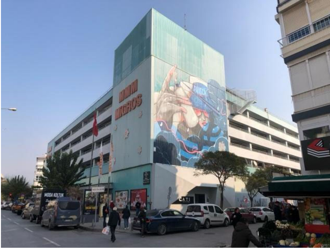
Figure 1. Çatı gallery, located on the roof-top of a parking garage in central Bostanlı, Karşıyaka Municipality, Izmir. Photograph: Torsten Janson.
