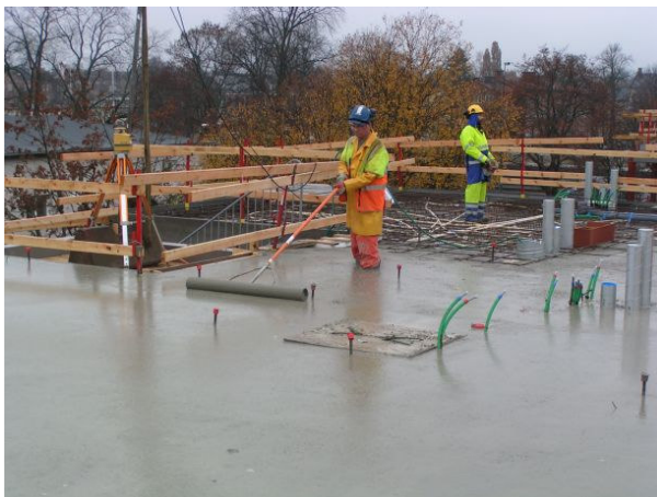
Figure 4.8 In Case 2 specially made top formwork was utilised in combination with SCC in order to achieve lower heights for slopes for drainage gutter. Note that the major part of the slab area was possible to cast with one and the same type of SCC based on increased adaptation grade to SCC compared to Case 1.
