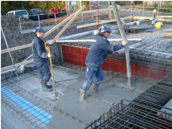
Figure 4.4 Casting of slab using SCC.
