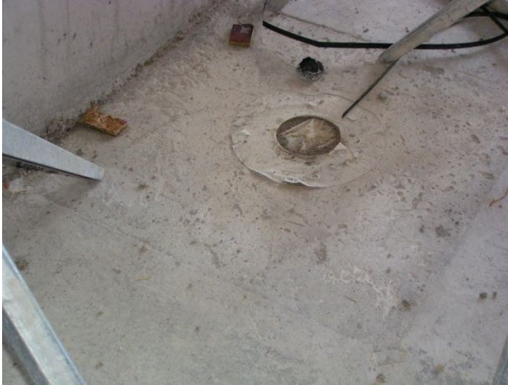
Figure 4.7 Example from Case 4 showing slope for drainage gutter in wet room directly achieved by SCC and top formwork.
