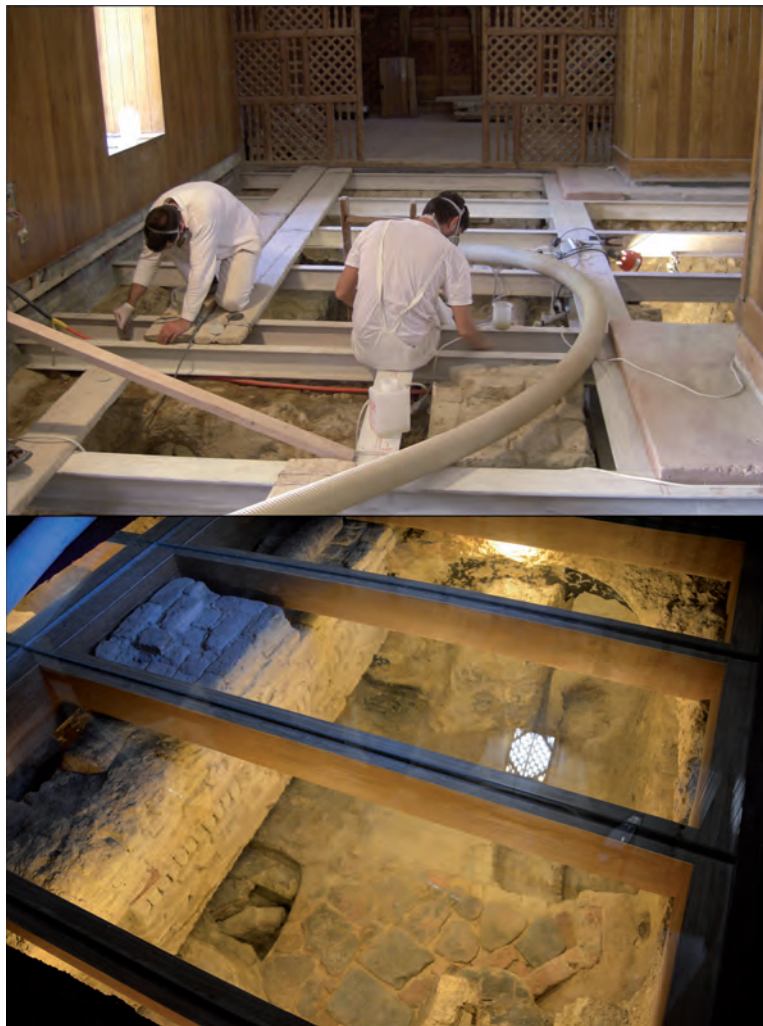
Fig. 17. Top: preparation of the steel supports for the glass floor (M. el-Antony); bottom: current glass floor of the Church of the Holy Apostles, displaying the excavated structures below (J. Blid).
