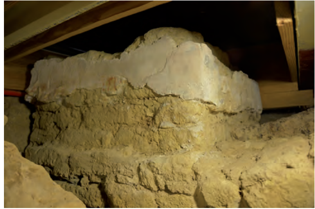
Fig. 10. Pier 2 dressed in stucco showing remains of paintings (J. Blid).
