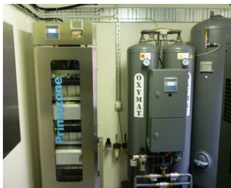
Figure 2 Inside view of the same container. Visible from the left - main PLC, ozone generator, and oxygen generator.
