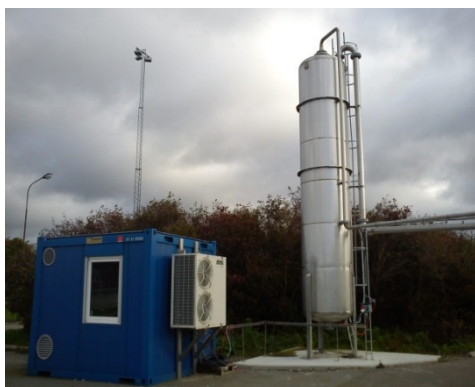
Figure 1 Outside view of the container and pressurized reactor installed at Klagshamn WWTP.
