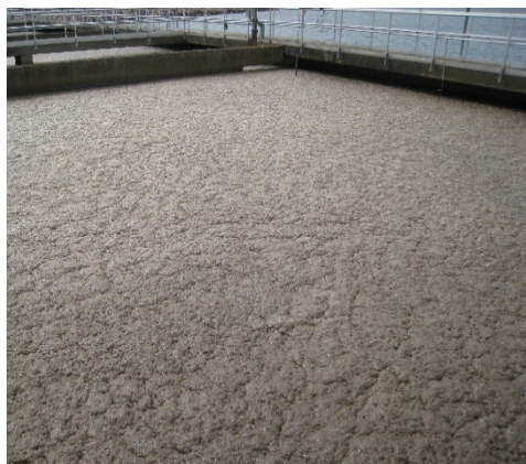
Figure 24 Aerated zone of untreated line at Öresundsverket WWTP
