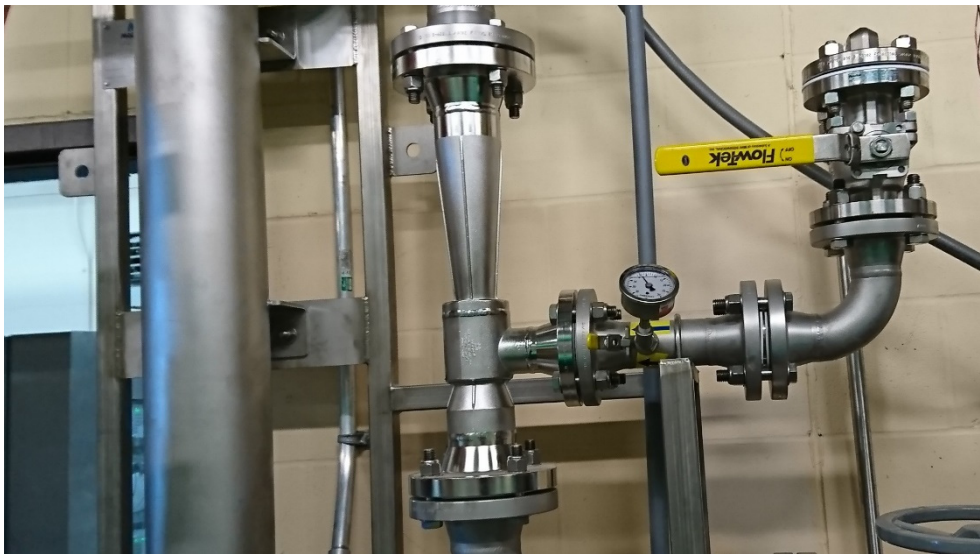
Figure 9 A venturi injector installed at a potable water plant in the US. The water flows upwards and ozone is injected in the port on the right hand side. Photo by Mats Cato (reproduced with permission).
