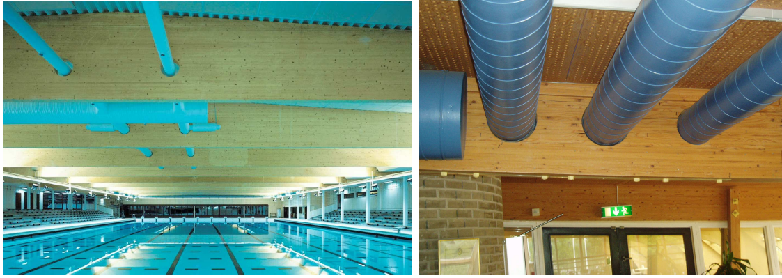
Figure 1.2: Examples of structures with glulam beams with holes. Indoor swimming pool, Västerås, Sweden (with permission for Martinssons Trä AB) and Restaurant Ideon, Lund, Sweden.
