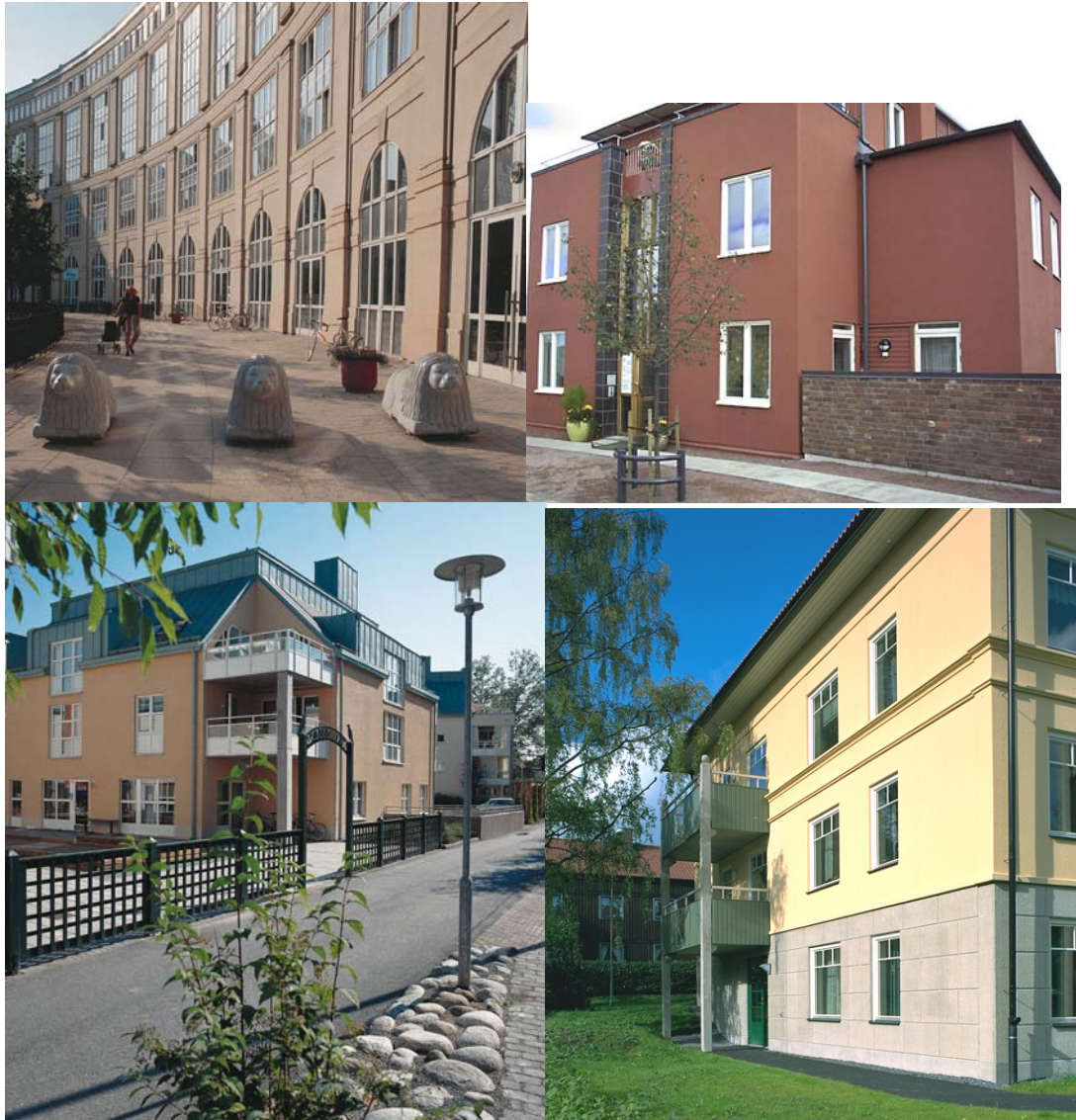
Figure 3.11 Examples of façade designs of modern Swedish precast concrete dwelling buildings. Top left: Stockholm, 'The Arch of Bofill'. Concrete surface similar to sandstone achieved by washing the fresh coloured concrete. Top right and bottom left: Both Stockholm. Special 'joint free' sandwich element with lightweight aggregate in outer panel. Bottom right: Frösön, Jämtland. Painted elements with surface structure similar to rendering and joints used as design element. Bottom right with permission of SCF Betongelement AB, Strömsund, Sweden, all other with permission of Skanska Prefab AB, Malmö, Sweden.
