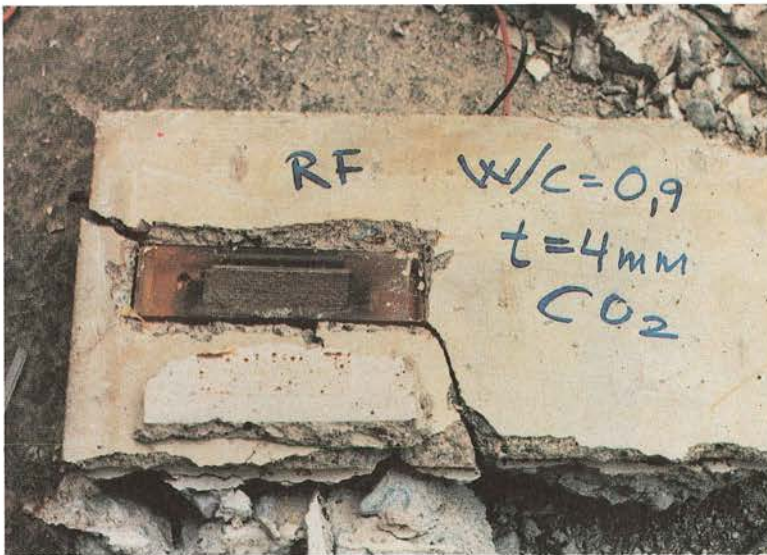
Photo 32. Corrosion cell in Series 3, KC6-78 which had been in carbonated concrete and then been subjected to wetting to study the cell current as a function of the relative humidity and temperature.
