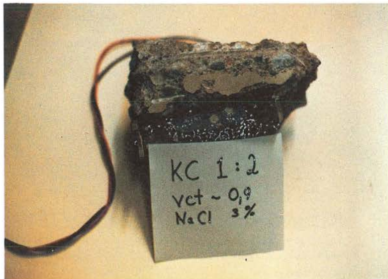
Photo 10. Corrosion cell after exposure to a 3% NaCl solution for about 60 days. A large quantity of corrosion products can be seen with the naked eye on the entire cell, particularly on the anodic areas. Concrete quality KC1-76, W/C approx. 0.8, concrete cover 7 mm.
