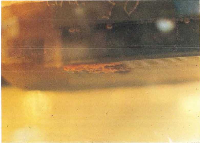
Photo 7. Close-up of corrosion cell in preceding photo.
