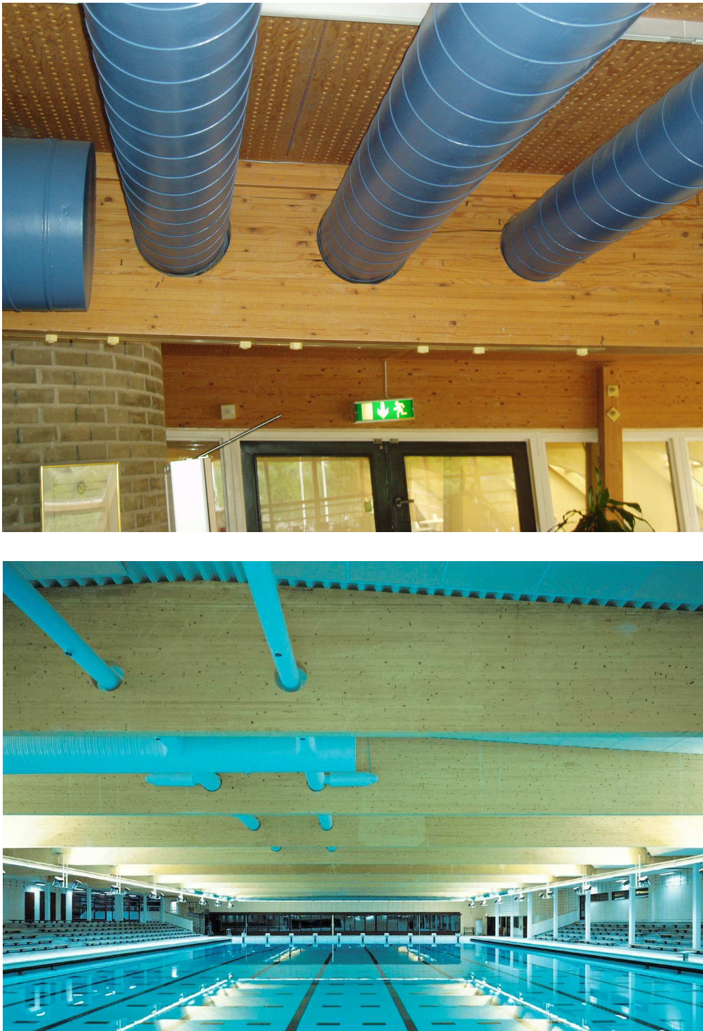
Figure 1.1: Examples of constructions with glulam beams with holes. Top: Restaurant Ideon, Lund, Sweden. Bottom: Indoor swimming pool, Västerås, Sweden (with permission from Martinsons Trä AB).
