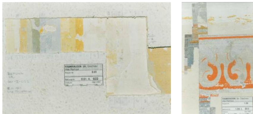
FIG 1: Exposed historic paint layers of a rectory of the 16th century in Haimhausen in greater Munich (Picture: Klaus Klarner, conservator, Munich)
