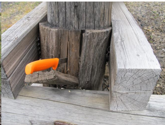
FIG 5. Decay in wood above soil contact is in areas where precipitation can penetrate into the wood, e.g. end grain and cracks.
