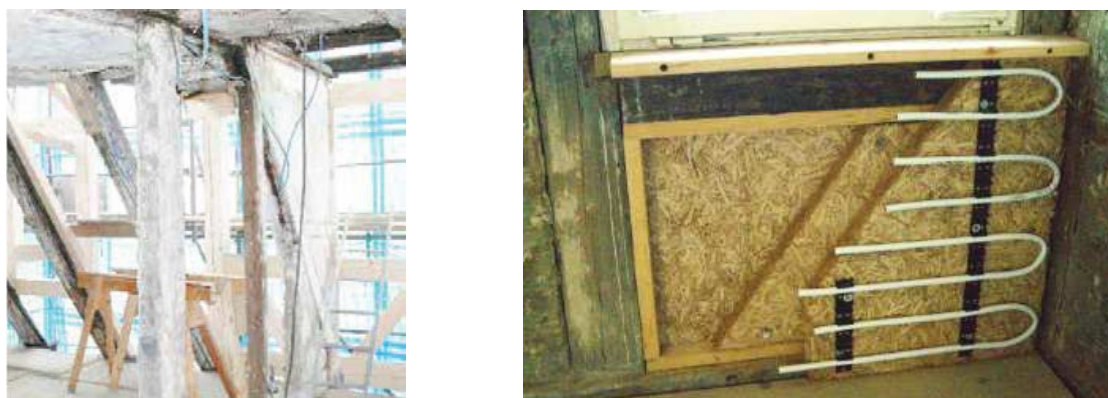
Fig. 2. Condition of the wooden framework before restoration (left) and scheme of the insulation (right), pictures by Alexandra Fritsch.
