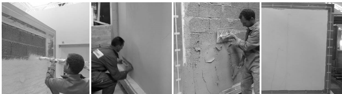
FIG. 2 – Application of renderings.
