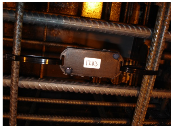
FIG 4. The RFID-tags were fixed by using plastic stripes looped around reinforcement bars.
