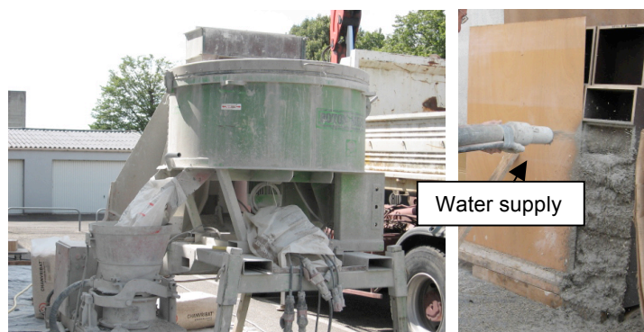
FIG 1. Implementation by spraying
