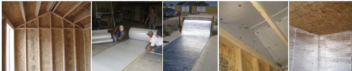
Figure 2: Left to right: uninsulated hut interior without ceiling, non-reflective insulation installed on the roof interior of Huts 2 and 3, reflective insulation installed on the walls of Hut 3 with ceiling installed.
