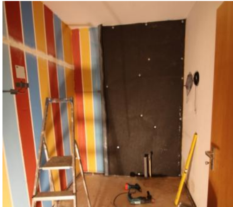
FIG 2. Interior view of the experimental building with the east and south walls with color swatches and some already mounted adhesive mat.
