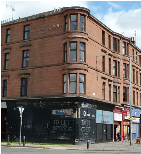
FIG 1. The wall being monitored is the west facing wall of the top floor corner flat with a fairly open aspect and with monitoring equipment installed to the left of the bay window.
