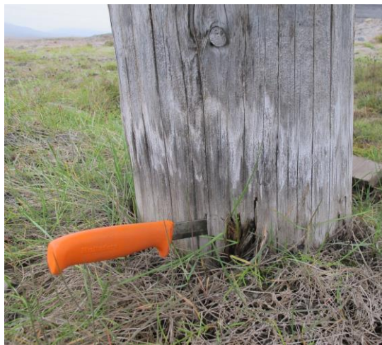
FIG 4. Decay damages were commonly found where the wood is in soil contact.
