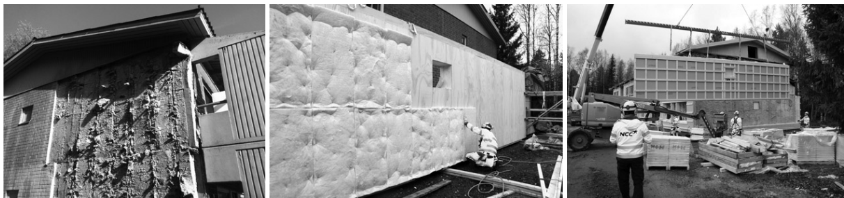
FIG 2-4. The façade retrofit started with the removal of redundant structures and an uneven inner concrete surface was revealed. A thin layer of thermal insulation was added as an adjustment layer to the prefabricated timber based façade elements prior to assembly. TES-elements were finally assembled directly onto the existing building, thus forming a new façade. The cladding was installed on site. Image to the left: Simon le Roux. Images 3 and 4: Jaakko Kallio-Koski M3 Architects.
