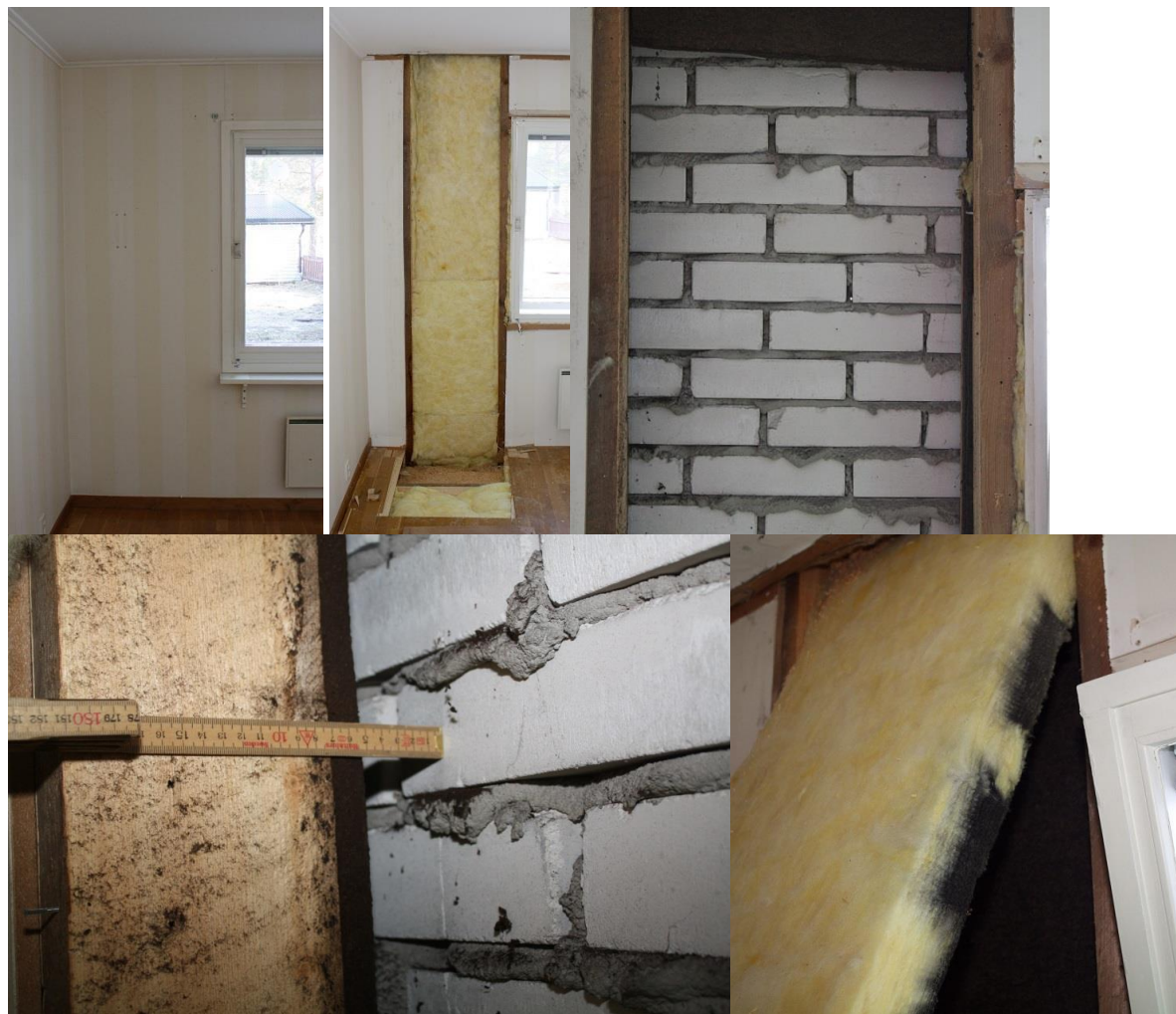
FIG 4. The wall investigation of house 1. It is dirty in the outer parts from the outside asphalt impregnated board but without apparent moisture damages.
