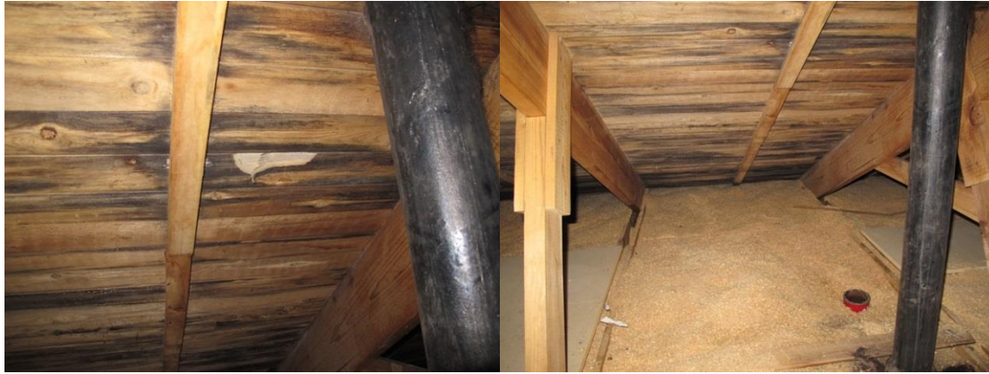
FIG 5. Mould growth in the cold attic of house 13.
