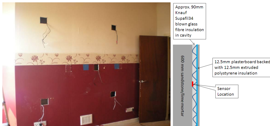
FIG 3. Interior sensor locations on west facing wall: temperature, relative humidity and moisture sensors are fixed to the internal stone face in the five locations where plasterboard has been cut away.
