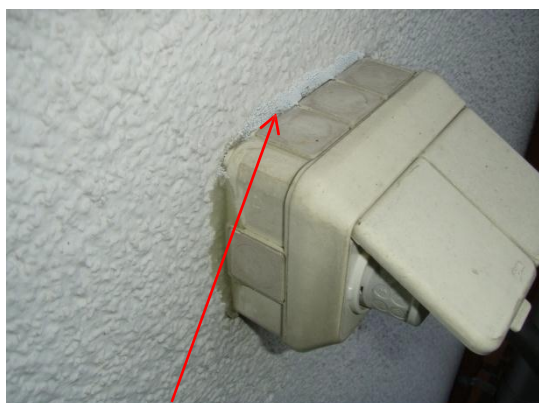
FIG 6. Poor joint at electrical service
