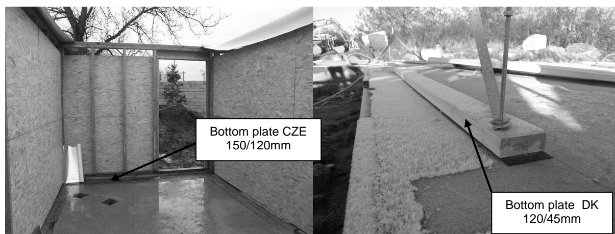
FIG 1. Total view on the wet wall of Czech study case (left), Bottom plate under weather condition in Danish study case (right)
