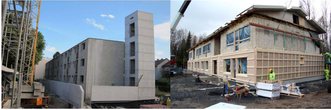
Figure 1: Left: Dismantled structure of Munich demonstration with new elevator shaft (Picture: Lichtblau Architects). Right: Oulu demonstration during assembly of prefabricated TES elements (Picture: Simon Le Roux).
