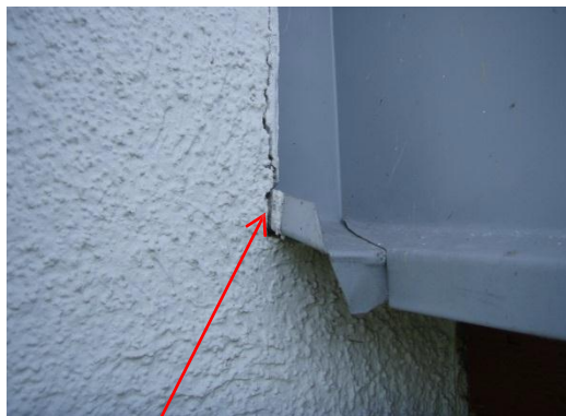
FIG 2. Leaking at the window sill
