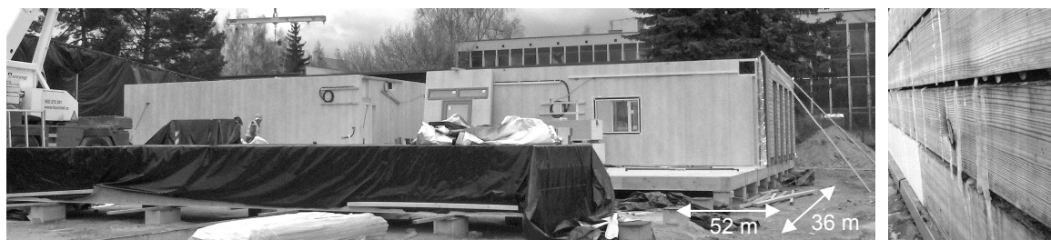
FIG 1. Prefabricated timber structure (left); northern facade with the freezing condensate (right)
