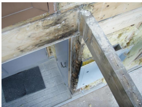
FIG 3. Extensive rot and mildew damage
