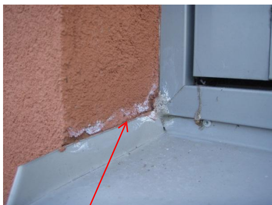
FIG 5. Poor joint at window sill
