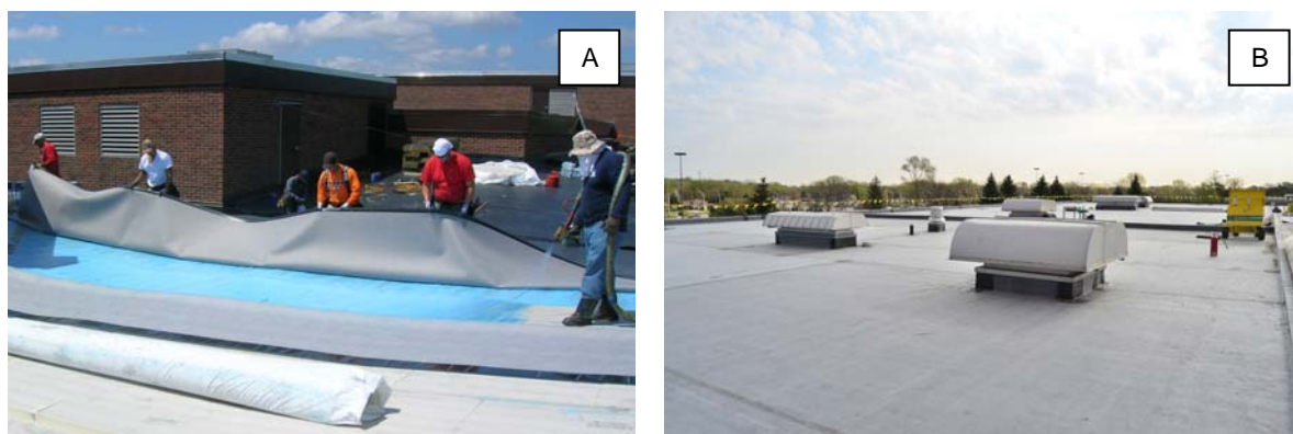
FIG 2A -B. Roofing crews set the 90-mil EPDM into the full coverage two component spray polyurethane adhesive, which will be rolled into place with a 90 # (41 kg) water roller. Note the two layers of insulation with offset joints and the roof edge sheet metal installation on the roof edges beyond. In the right photo the 45-mil vapor retarder has been installed, and the raising of the roof curbs and edges, replacing roof drains, and modifying mechanical equipment can take place.
