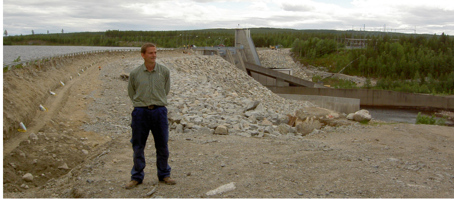
Figure 24. Hällby dam during the reinstallations of electrodes in 2005. The top of the right dam crest is excavated and new electrodes are being placed out, every second being a non-polarisable (white bags). The downstream slope has been reinforced with additional rockfill. In the background are the spillways, the intake to the power station (high building) and the left embankment dam. Author in front.
