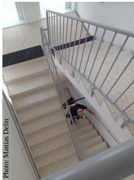
Figure 12. The stairwell in the Ideon experiment.
