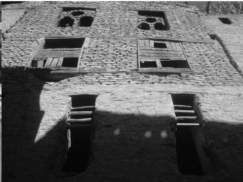
Mud brick vernacular buildings in the oases can be up to four stories high.
