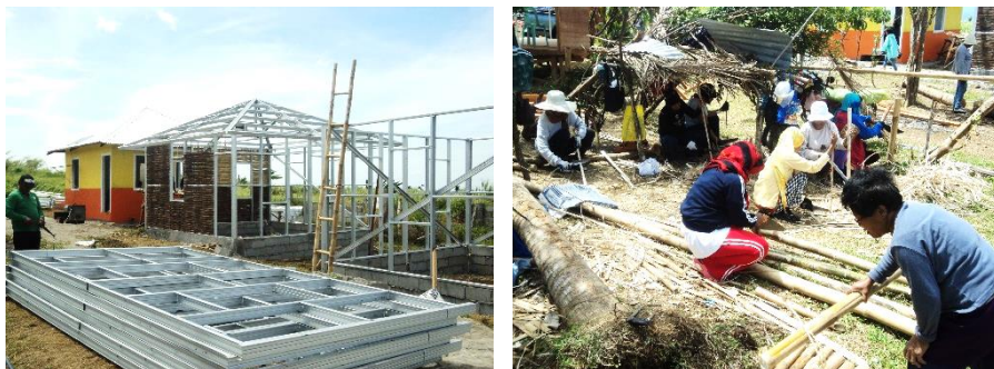
Figure 4.12 Housing solution and women working with bamboo, We Effect's pilot project in Barangay Dolores, Ormoc. The images show the construction method and women cutting, preserving and preparing bamboo for the walls. Pictures: by the author, March 6, 2014
