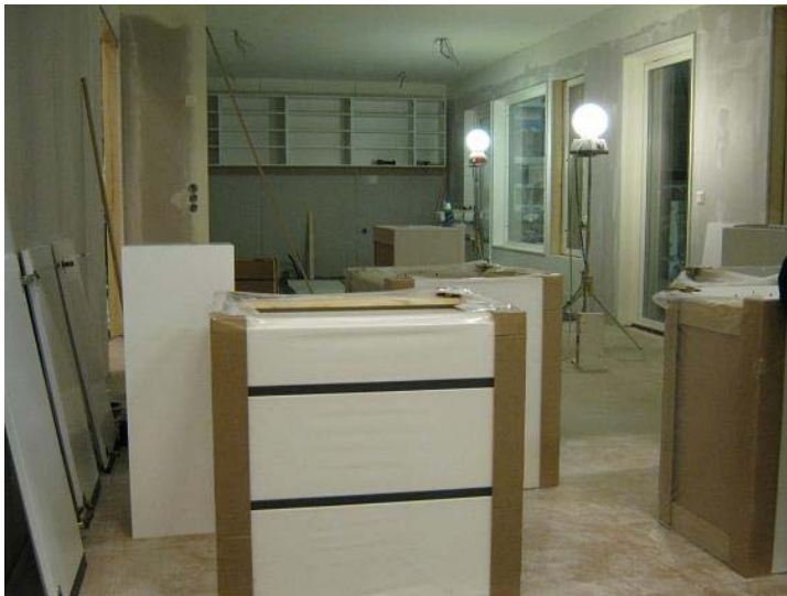
Figure 1: Kitchen installation in a volume element
