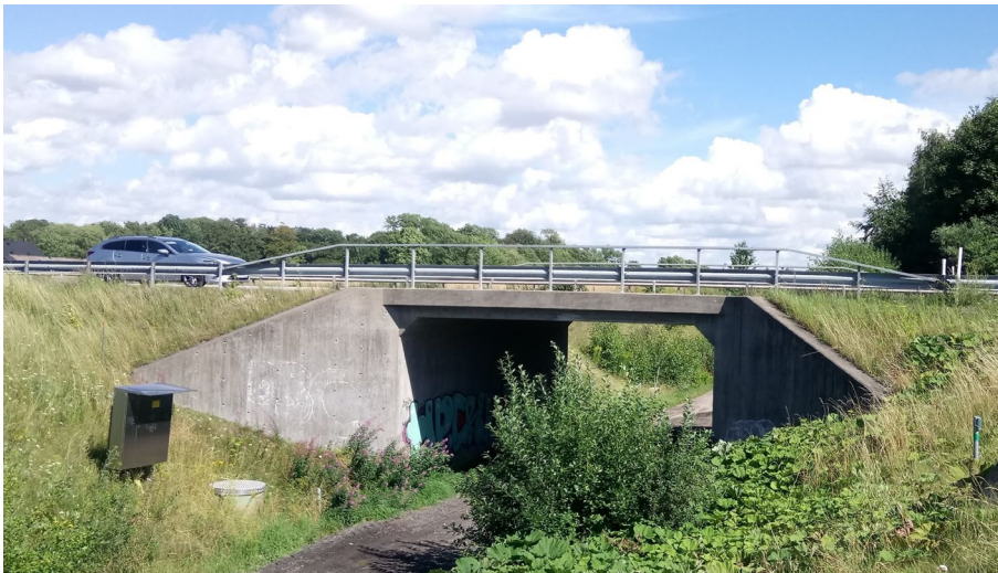
Fig. 2.1. A portal frame bridge.
