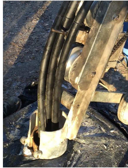
Figure 5 – Installation of single and double U-tube ground collectors in the 200-m deep borehole for in-situ tests.
