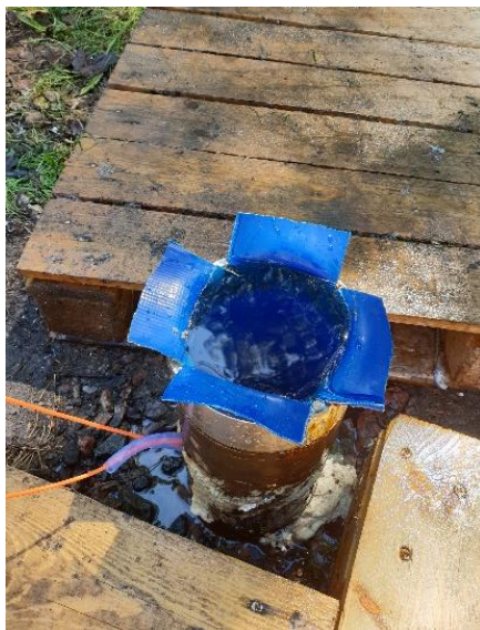
Figure 6 – Installation of the coaxial collector with a flexible outer pipe in the 200-m deep borehole for in-situ tests.
