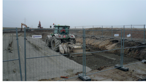
(b) Mixing binder with the original soil.
