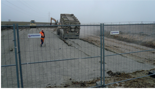
(a) Spreading out binder material.
