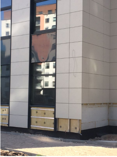
Figure 3: Example of a ventilated façade on a building in Riga, Latvia, (a) during construction with exposed insulation and railings (b) over the entire façade of a high rise building
