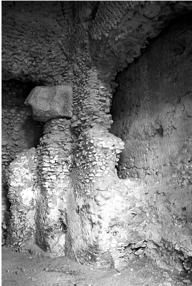
Fig. 4. One of the chambers in the tomb of Sempronius Atratinus at Gaeta, showing double interior walls with an intermediate space (photo Henrik Gerding)
