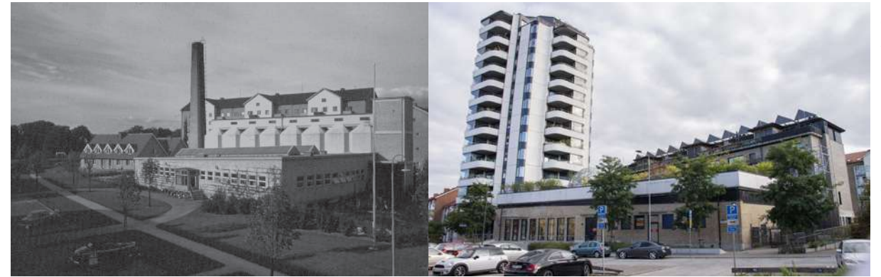
Greenhouse is located in the same spot in Augustenborg as the former heating station and common laundry room. It's a conscious decision, well in line with MKB's strategy of urban acupuncture - "lifting" an area through individual incision investments.
