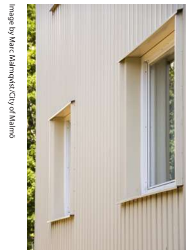
When insulation and a sheet metal facade was added to the rendered houses in the late 70s, the windows were set deeper than before, changing the appearance.
