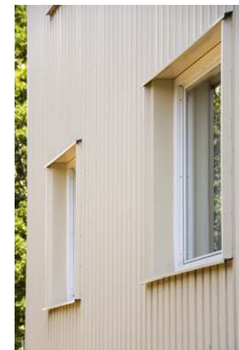
When insulation and a sheet metal facade was added to the rendered houses in the late 70s, the windows were set deeper than before, changing the appearance.
