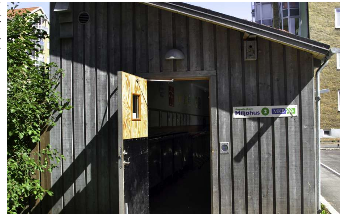
There are 13 recycling houses in the residential area, some with or some without windows. Here, residents can separate packaging made from paper, plastic, glass and metal as well as newspapers and food waste.
