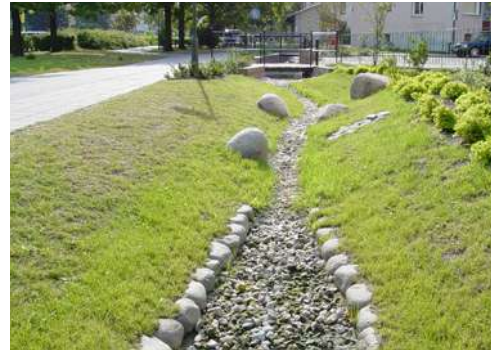
Image 7. Stormwater swale along Lönngatan. Image by Ulf Thysell. The gutters here were given lattice covers, rather than being open, making the stormwater system less visible in the urban environment, see Image 8.
