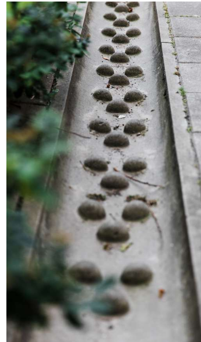
An example of local innovation from Augustenborg: the so-called onion gutter in the open stormwater system. Image by Sanna Dolck
