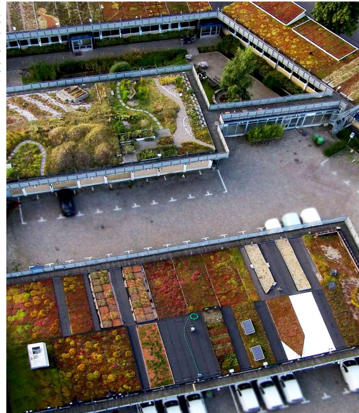
The roof garden is not only a research facility, but also allows displays and testing of different types of green roof.
