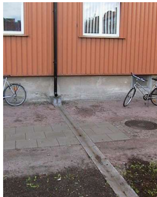
Image 2. The drainpipe and gutter in stage 1, southern section. Image by Lars-Erik Widarsson and Ulf Thysell.
