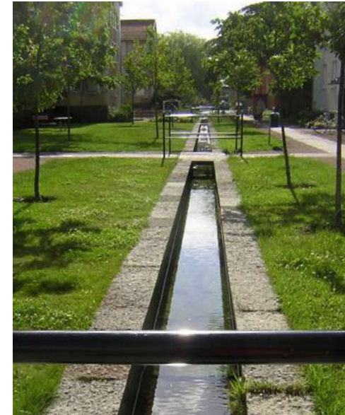
In Augustenborg's sustainable urban drainage system, the water travels slowly through canals, ditches and ponds, through greenery and surfaces that can withstand floods.
