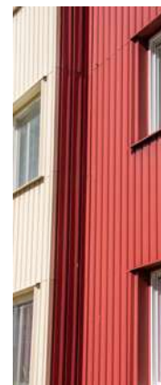
A new facade of corrugated metal cladding
