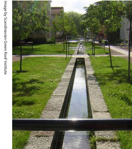
In Augustenborg's sustainable urban drainage system, the water travels slowly through canals, ditches and ponds, through greenery and surfaces that can withstand floods.
