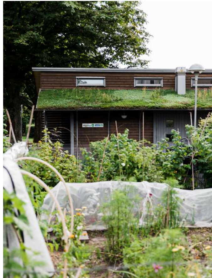
Augustenborg has become a green city district, which is welcomed by the residents and strengthens biodiversity. This is one of the district’s 13 recycling houses. Image by Sanna Dolck
