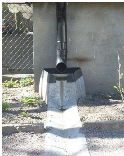
Image 2. The drainpipe and gutter in stage 1, southern section. Image by Lars-Erik Widarsson and Ulf Thysell.
