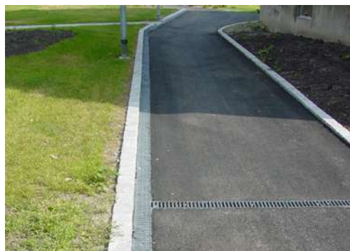
Image 8. During stage two, which developed the northern section, the open gutters were replaced by latticed gutters, and the gravel with asphalt. Image by Ulf Thysell
