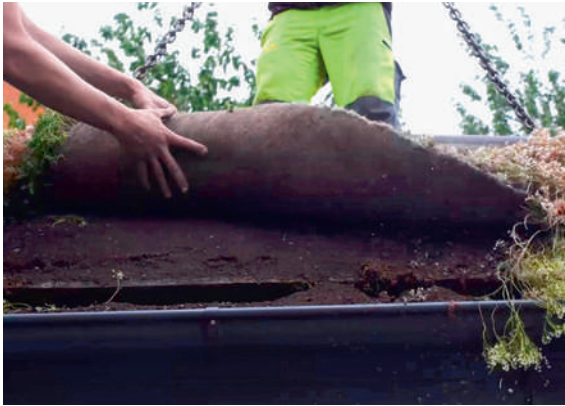
This is how a finished sedum carpet looks from underneath. Image by Jonatan Malmberg.
