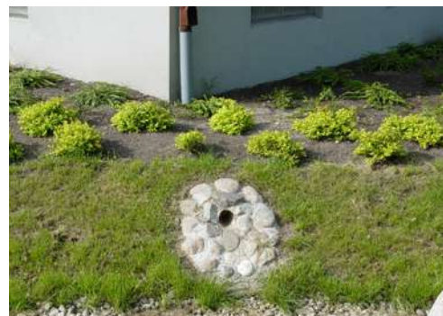
Image 9. In stage two, the northern section, it is less obvious that the drainpipe deposits its water above ground. Image by Ulf Thysell.
