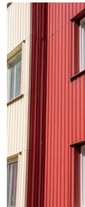
A new facade of corrugated metal cladding
