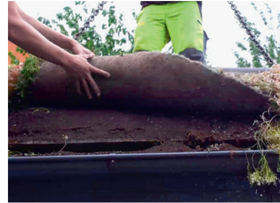
This is how a finished sedum carpet looks from underneath. Image by Jonatan Malmberg.
