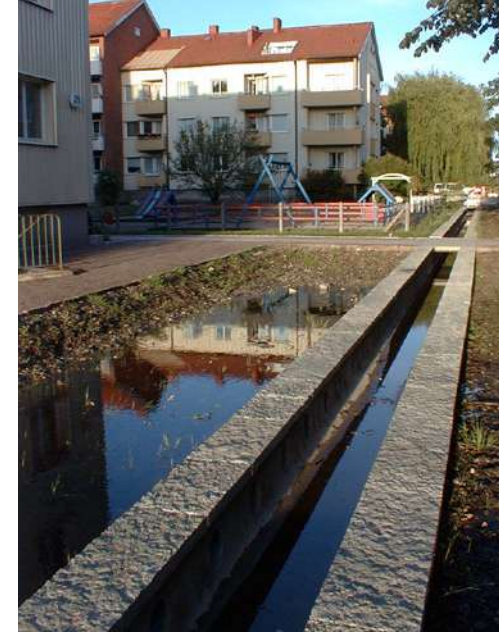
Image 3. The '50s-style concrete canal. When the picture was taken in 2002, railings had not yet been installed at the canal crossings. Image by John Dolocek.
