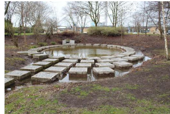
Image 5. At the end of the system a large pond slows the water's journey. An overflow mechanism that leads into the pipe network in the street beyond is visible at the far end of the pond. The picture was taken in 2016 shortly after the surrounding vegetation was cleared and cut down. Image by Stefan Billqvist.
