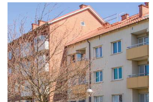
Some of the balconies in the area were given a new look during the 1980s.
