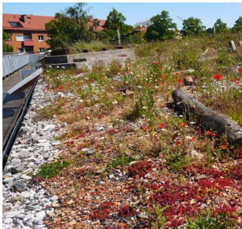
The roofs are constantly evolving. This is the so-called ruderal roof, photographed every ten years. Some of the limestones were later changed for a substrate that better retains water.
