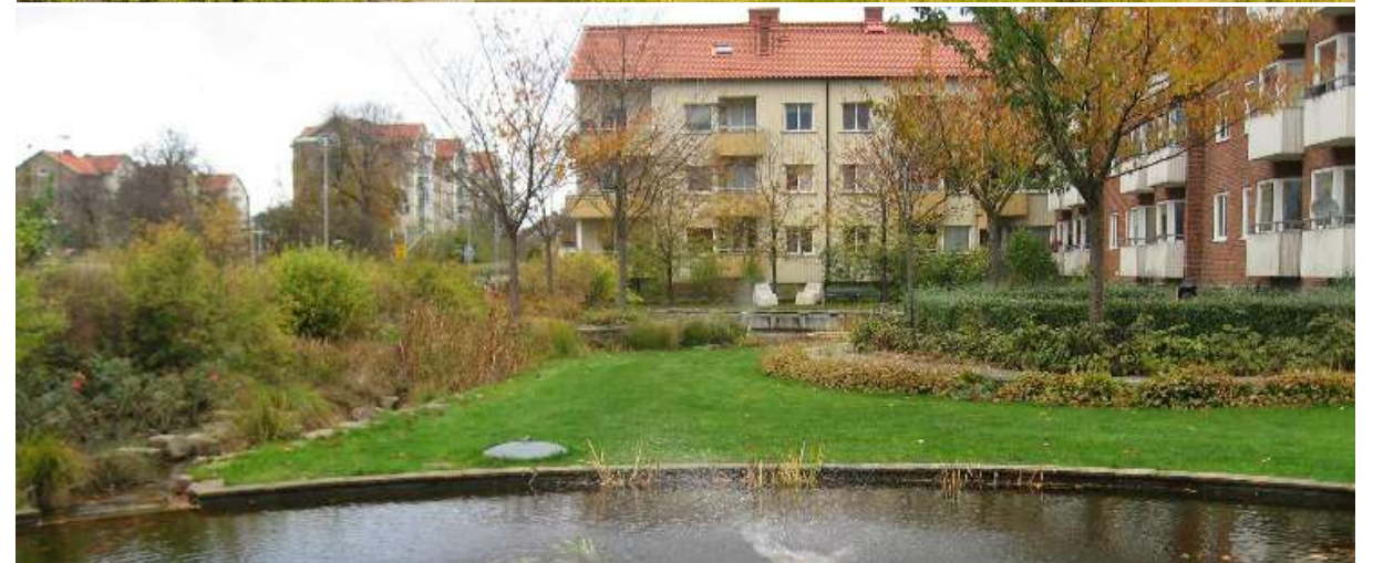
Image 10. The pond at Södra Grängesbergsgatan. A. Newly built pond 2002, image by John Dolocek. B. The pond a year later, image by Ulf Thysell. C. Redesigned pond in 2012 which had the same holding capacity but was differently designed and had a pump to circulate the water, image by Leif Runeson.
